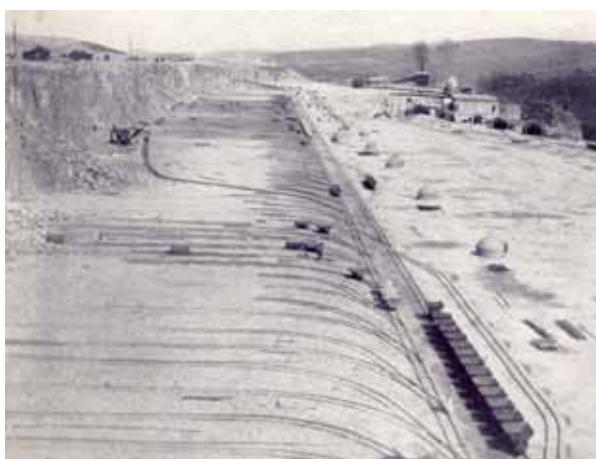
Figure 3.30 Tunstead Quarry, Buxton replaced up to twenty other operations between the wars and continues today as a technological leader. The transition between hand- (foreground) and machine-filling (distance) is shown here in 1948. Although change has resulted in physical loss, almost every adaption has been recorded in an extensive photographic archive. © NSC collection
