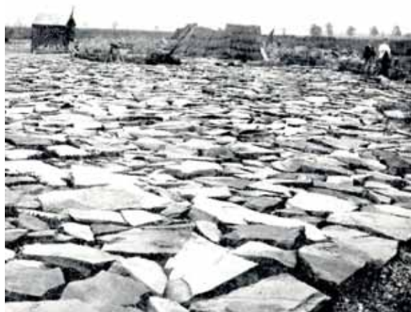
Figure 3.21 In order to split fissile limestones for roofing as here at Collyweston, Rutland, blocks ('logs') were traditionally left outside to over-winter using freeze-thaw processes. © Greenwell and Elsdon
