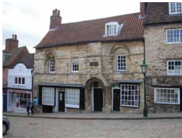
Figure 3.6 Even where stone was readily available, its post-Roman use was largely confined to churches, bridges and defence; the 12th-century Jew's House at Lincoln is exceptional and probably the oldest still occupied stone house in England. © Ian Thomas
