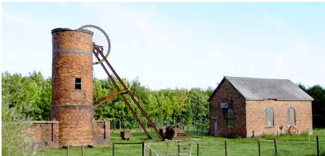
Figure 4.8 Unusual headgear built into brick tower at Western Fan shaft, Western Derbyshire. © Ian Castledine
