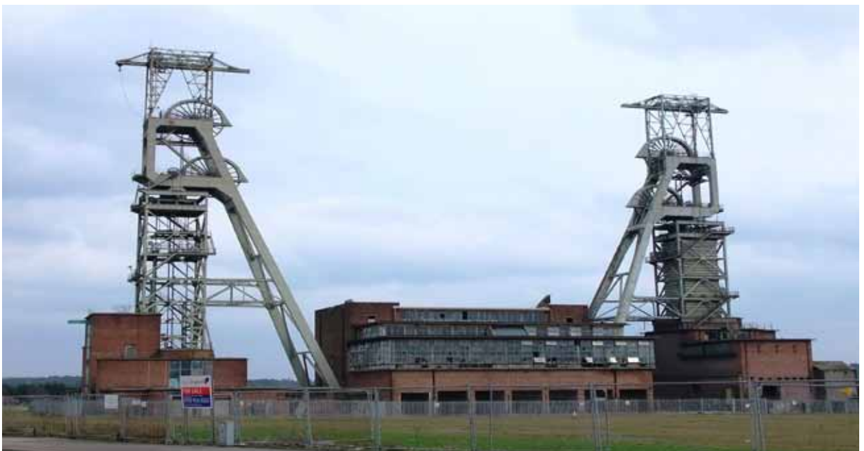
Figure 4.3 Double headstocks at Clipstone Colliery, Nottinghamshire. Koepe Headgear and winder. © Ian Castledine
