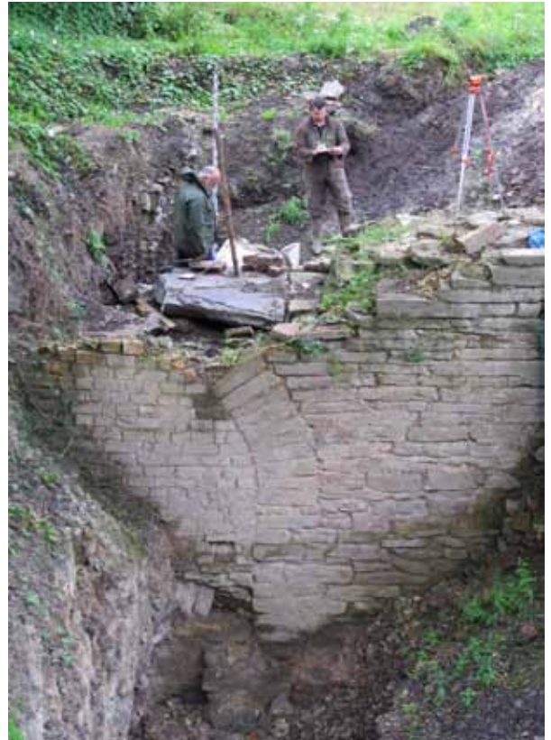
Figure 4.12 The two lower storeys of the 1791 Serridge Newcomen Engine House were hidden below the surface and their existence entirely unsuspected prior to SGMRG's ten-year programme of excavation and conservation.
