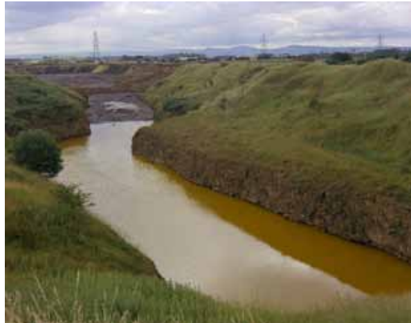
Figure 3.26 Geology plays a vital role in defining quarry format. Extraction of basaltic andesite along the Cleveland Dyke is an extreme example. The feature runs for c.370km from Mull almost to Whitby. Workings crossing the North Yorkshire Moors are typically 22m wide and 30m deep as at Coatham Stob. British Geological Survey CP15/061 © NERC 2015 All rights reserved
