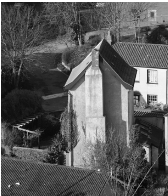
Figure 4.2 This Newcomen engine house at Brislington, in the Bristol coalfield, has national significance as the UK's oldest intact engine house. It is mentioned in accounts of 1740 that confirm that the structure, which contained an engine with a 28" cylinder, was built c.1739. © Steve Grudgings
