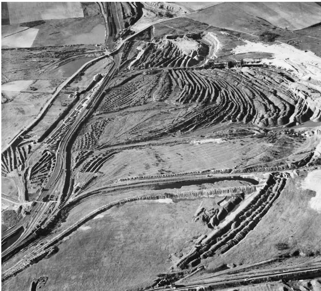
Figure 5.6 Aerial view of opencast Ironstone Works at Crosby Warren, Scunthorpe, 1950. Although fragments of what is visible in this photograph survive, most has been obliterated by later working. © Britain from above EAW028901
