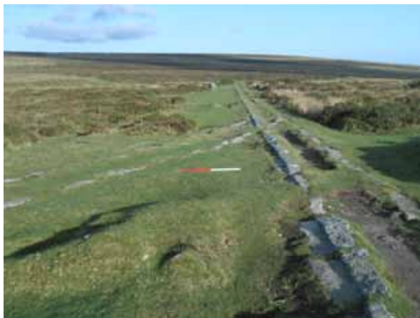
Figure 3.35 Haytor Quarry, Dartmoor displayed a unique and innovative means of transport in 1820 utilising granite 'rails'. © Phil Newman
