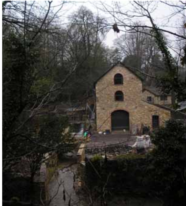
Figure 3.24 Compared with other mineral workings, water power was rarely used to crush stone. Hapsford Mill, Frome, Somerset operating c. 1900 was an exception. © Ian Thomas
