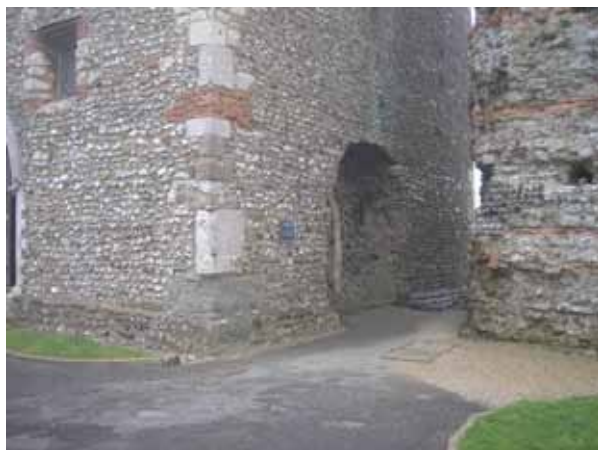
Figure 3.5 For several centuries after the Romans departed, their buildings became virtual quarries. Depleted Roman lighthouse (right) and adjacent Saxon church (left), Dover Castle. Ian Thomas
