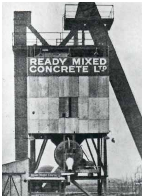
Figure 3.36 Although several thousand plants making coated roadstone, concrete products or ready mixed concrete (RMC) have operated in England, it is very doubtful if a single example has been recorded, let alone preserved. The first RMC plant started up at Bedfont, Middlesex in 1930, is seen here c.1950. © CEMEX
