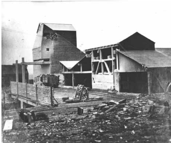
Figure 3.28 Timber and corrugated iron plant buildings at Cliffe Hill, Leics, typical of the period up to the 1970s. Like their more recent counterparts, planners will normally insist on complete removal on closure. © NSC collection
