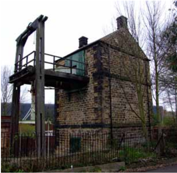
Figure 4.9 Newcomen engine house at Elsecar Yorkshire which still contains the engine for which it was originally built. © Ian Castledine
